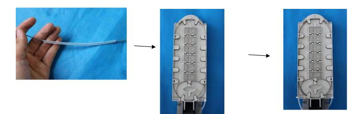
6.3.9 Processing the fiber splice, fix on splice sleeve holder, and coil the remain fiber into the fiber storage plate.
