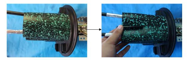
6.3.7 Proceed the heat shrink process for the cable and heat shrink tube, not let the fire close to the bottom of closure and the cable with foil paper.
