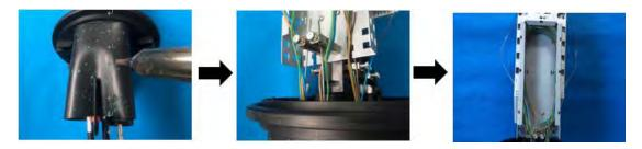
4.3.4 Put the required fibers of these two cables into buffering tubes, then put them into trays and fix them with cable tie. Manage the fibers in the tray and lead them through splice protectors to splice.
