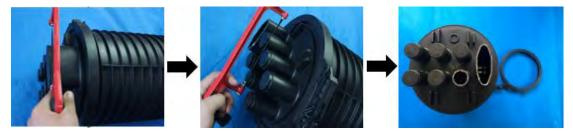
4.3.2 Use sand paper to polish the surface of the ports. Wrap up the heat shrink tubes, then pass the cut and uncut cables into the closure from the heat shrink tubes.
